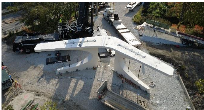
Construction continues at Ronan Park with pavilion installation.
