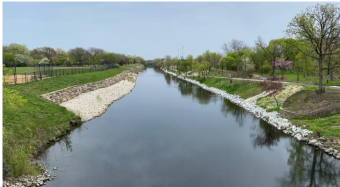
Riverbank restoration work at Legion Park improves habitat and connectivity.
