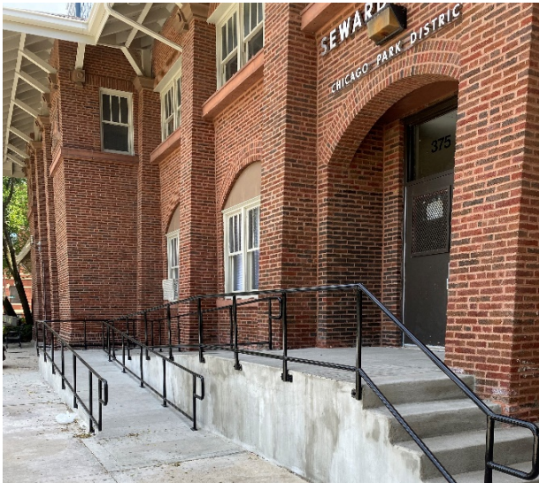
After significant fire damage, the Washington Park Field House was fully renovated in 2022 (above). The historic Seward Park Field House reopened in 2022 after $4 million of improvements to building envelope, interior and accessibility.
