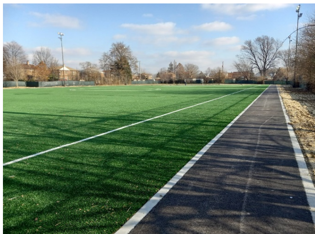
A new artificial turf soccer field and walking path was completed in Lawler Park in 2022
